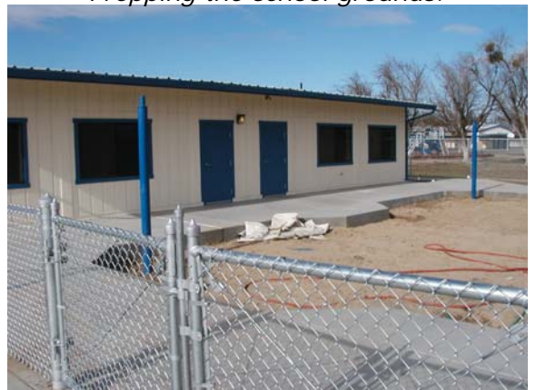
Building and concrete completed.
