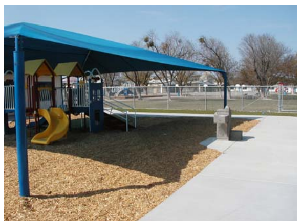
Play equipment and shade installed.
