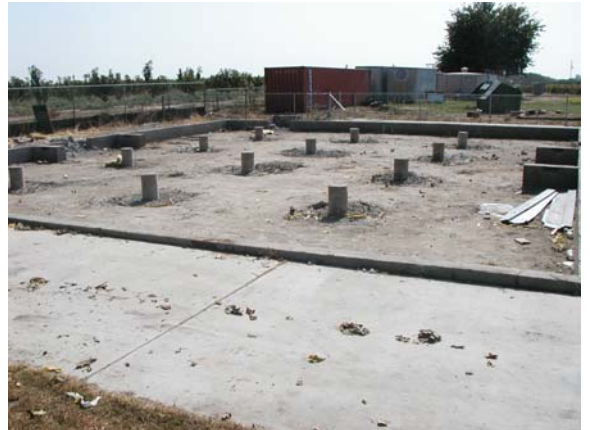
Prepping the school grounds.
